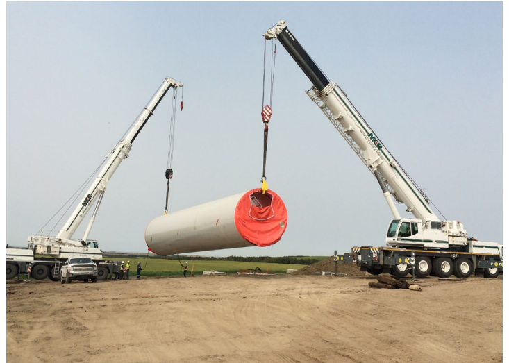
Turbine Assembly. Turbines are assembled and installed using cranes.
