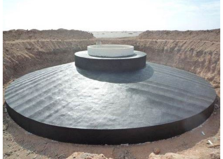
Turbine Foundations. Foundations for the wind turbines are constructed from concrete and steel.
