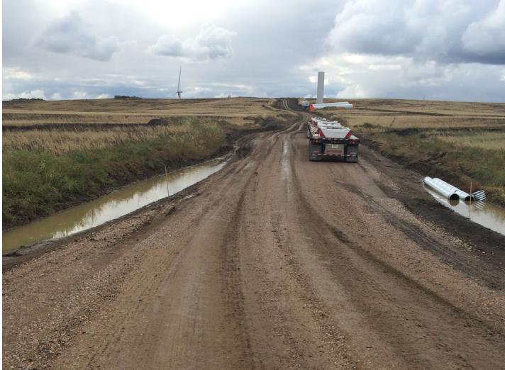
Civil Works. The ground area is prepared and construction of roads and laydown areas begin.
